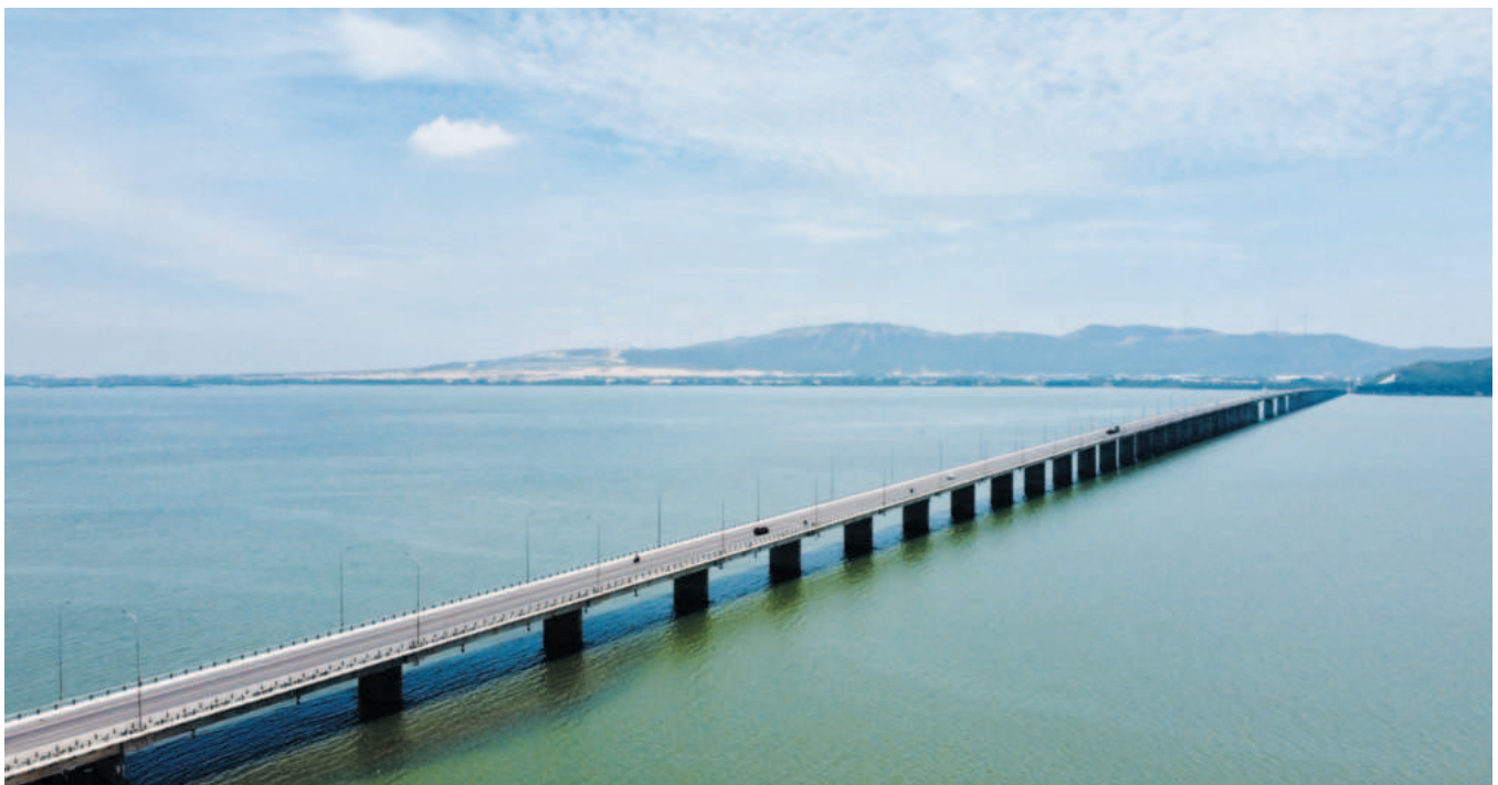
Thi Nai bridge is the longest bridge in Binh Dinh province
