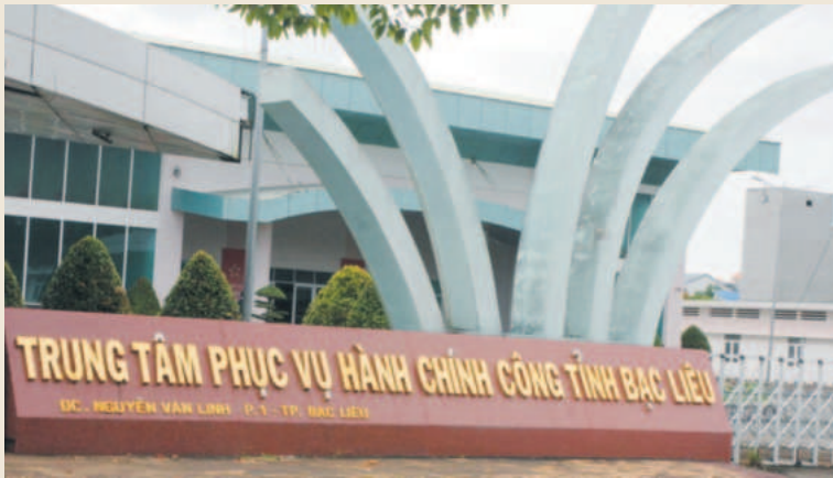
Bac Lieu Provincial Public Administration Service Center significantly improves the efficiency of administrative procedure processing for citizens
